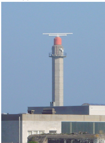
Figure 2: Radar scanner in Oostende
