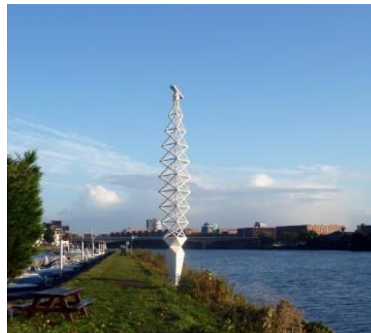
New radar scanner at the River Meuse
