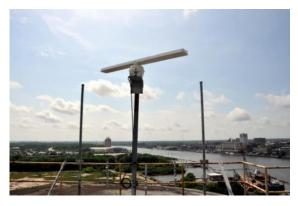
position and velocity of all objects on the river. Radar data are transmitted via DSL from harbor to the VTS display located at the building of Georgia Tech.
