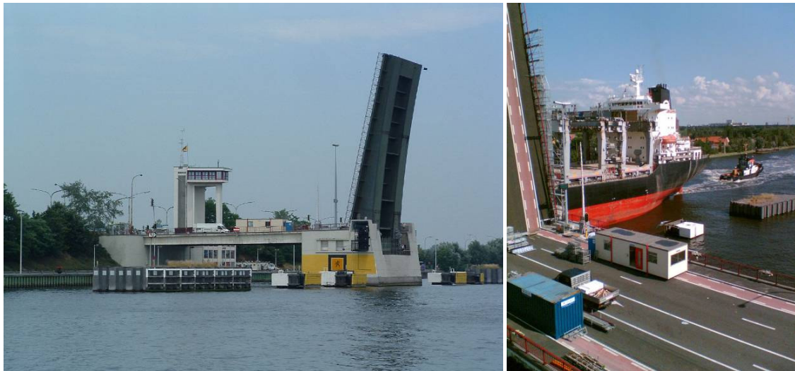
Figure 1: Zelzate Bridge over the Ghent canal, Belgium
