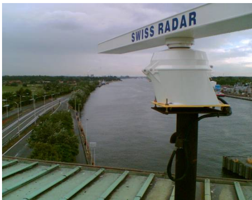
Figure 2: Radar scanner at Zelzate Bridge
