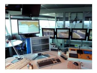
Thereby, a two-in-one display provides the overview as well as a detailed view of the lock entrance area at one glance.
