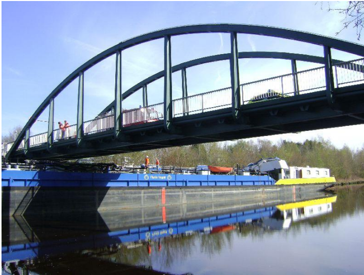
Cargo vessel after collision with bridge
