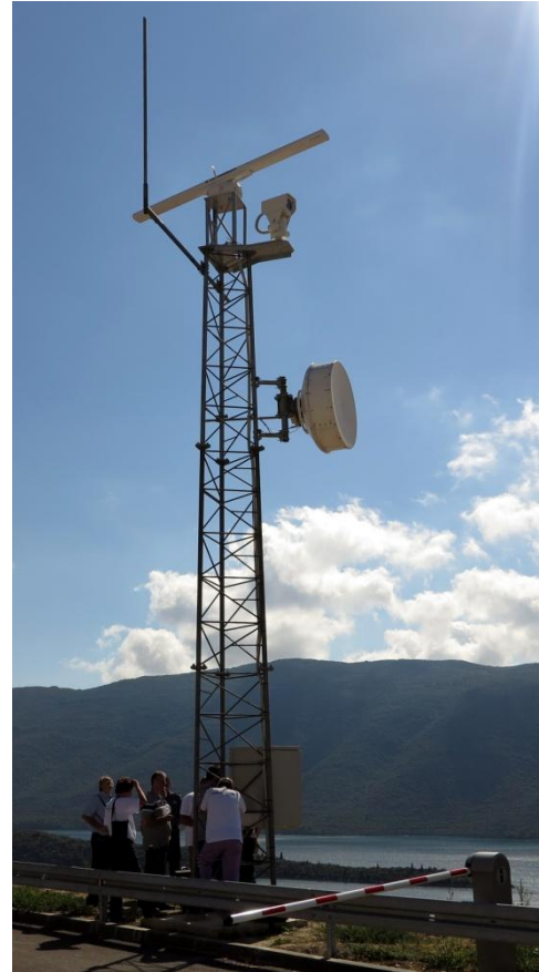
Approval of a radar/CCTV station
