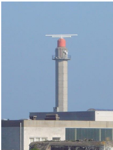
Figure 2: Radar scanner in Oostende
