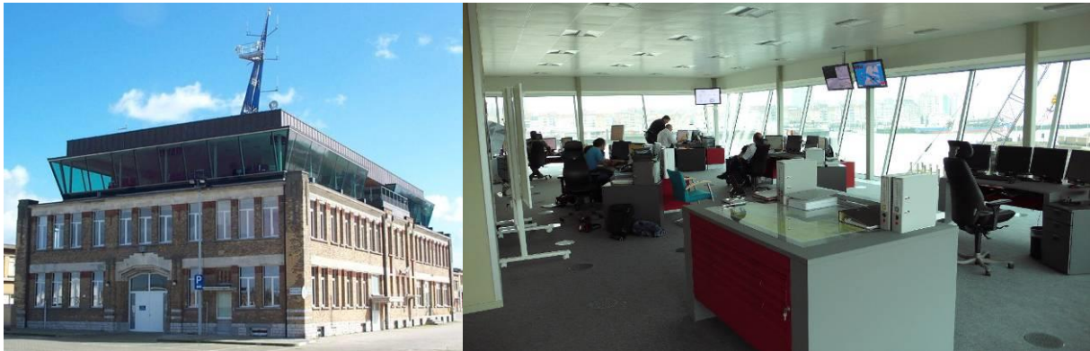
Figure 1: MRCC Oostende, control centre
