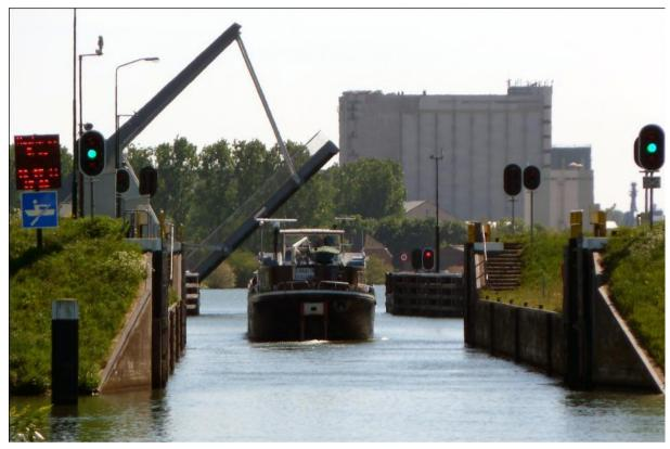
At the bascule bridge in Macharen, in the Province of North Brabant in the Netherlands, recently a new radar system was installed to monitor vessel traffic on arrival and departure to this bridge. The system uses two radar antennae as sensors, which are set up on pylons on both sides of the bridge. The display and remote operation of radars takes place in a control center about 10 km away, located in the control center of the lock Lith on the Meuse.
